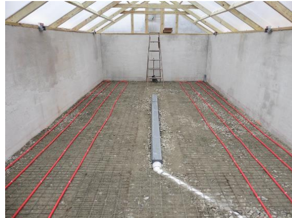
Figure 3. (A) Efficiency can be increased further if air is circulated through perforated ducts in a subfloor (left), (B) project included 4 independent zones of hydronic heating pipe (right).
